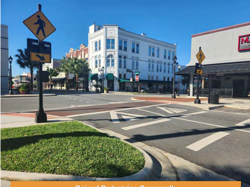
Raised Pedestrian Crosswalk
