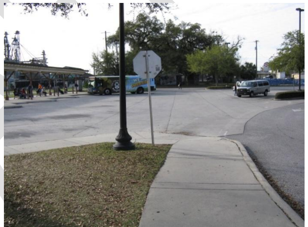
CURB RAMP TO PARKING AREAS
