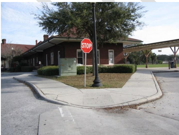
CURB RAMP TO PARKING AREAS (OPP VIEW)
