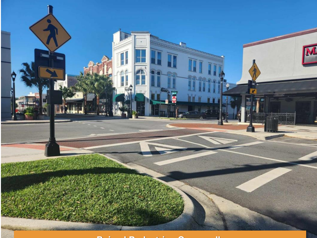
Raised Pedestrian Crosswalk
