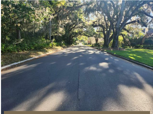
SE 5 th Street, west of SE 13 th Avenue, looking east
