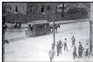
Courthouse on the Square 4
