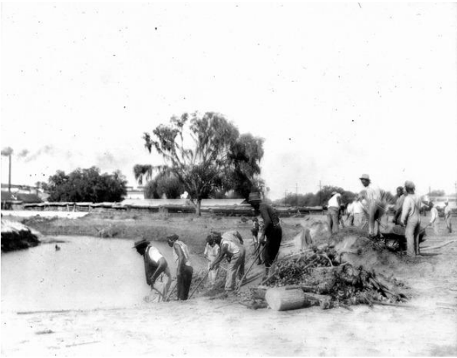
1935 photo taken during the construction of tennis courts (Source: Florida Archives)
