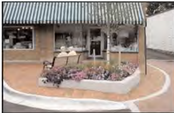
Bulb-outs extend out into the street to create a larger sidewalk area for pedestrians and a more narrow passage for cars. These areas can feature landscaping, trees and street furniture.
