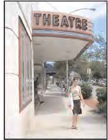
Rehabilitation and re-use of the Marion Theater is a key action step to immediately jump-start implementation.
