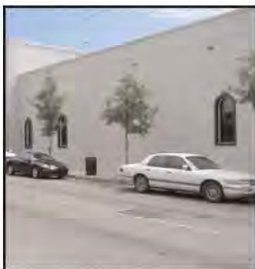
Long, blank walls are impediments to creating comfortable pedestrian environments.
