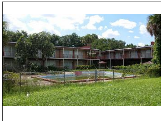
Dilapidated Motel - Ocala, FL
