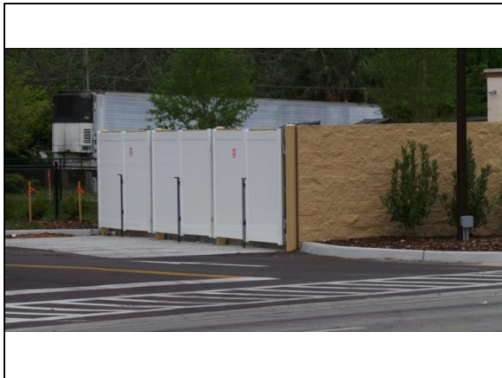
Recyclables and refuse collections, although necessary, need not be visible. Should either be located in the rear of buildings and businesses or in an attractive enclosure.
