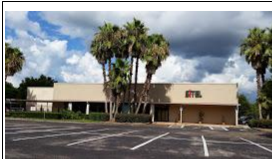
All utilities, service areas and mechanical devices should be screened from public view. If placed on a roof, an appropriately sized parapet should screen such appurtenances from view.
