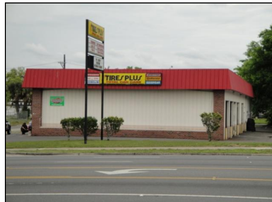
Vacant or void space walls should never face streets or roadways. Increases safety concerns for pedestrians.
