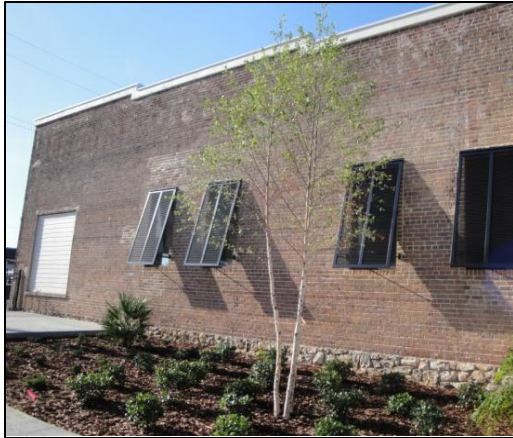
Security grilles should be integrated into the design of the building and should be unobtrusive when the business is open. Use of unbreakable glass or placing grilles inside of windows or doors is preferred.
